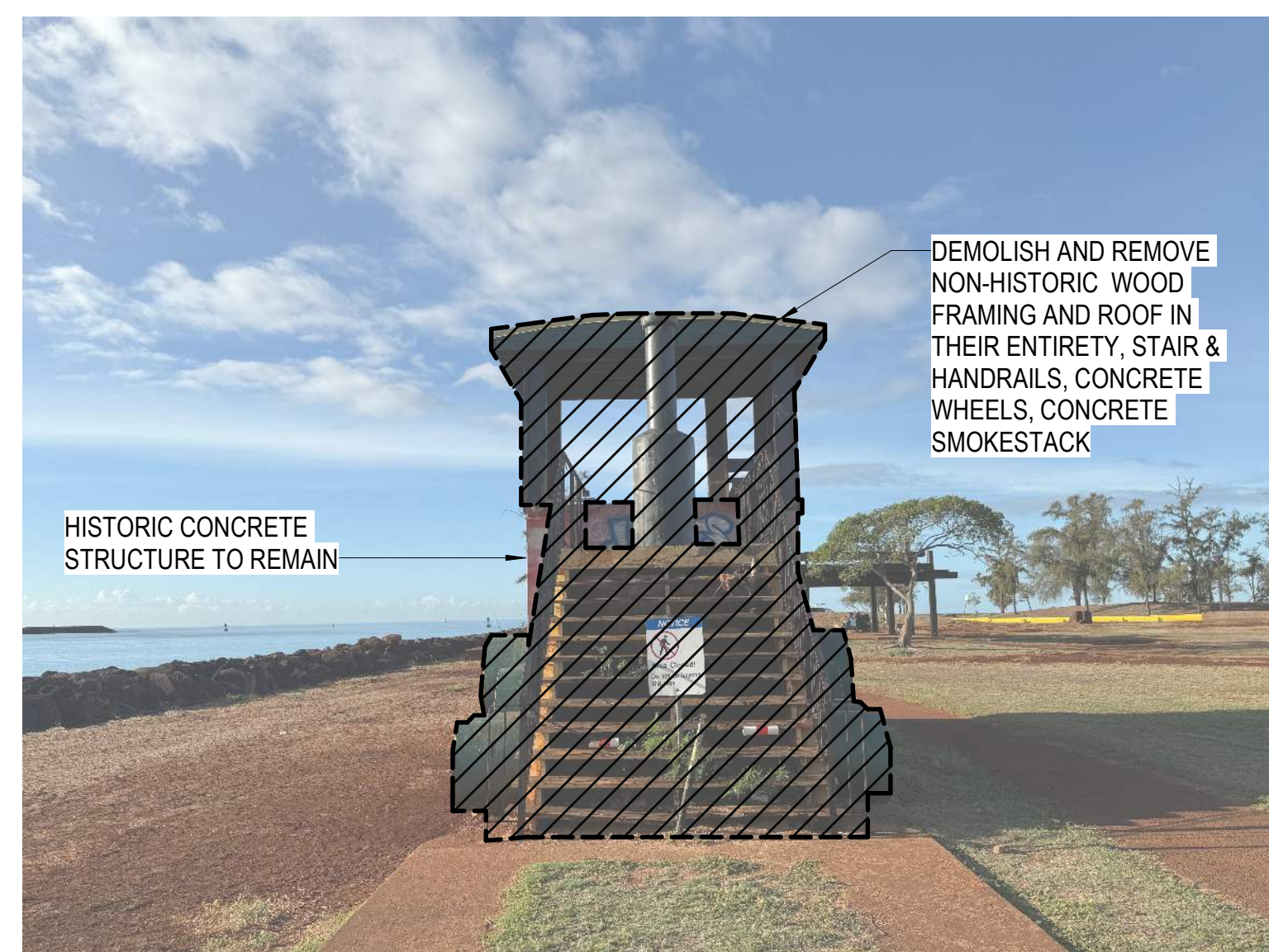
4 CABLE HUT (TRAIN)_NORTH ELEVATION (PHOTO) SCALE: 3" = 1'-0"
